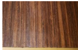
Plate 6. Installed Elaies guineensis Panels
